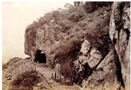
Tunnel under construction.
