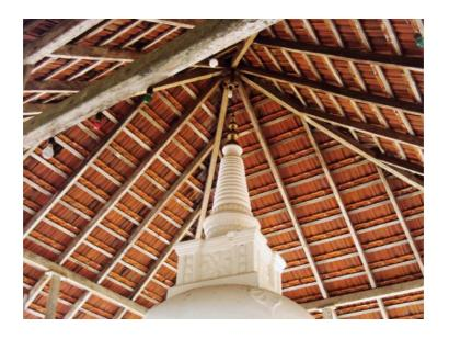
In contrast to the roof of Vatadage (which is generally circular in plan), that of the Kuludage is square in plan and supported by pillars at four corners. Pinwatte and Ahugoda however represent examples of kuludages of simplest design, while Nissankalata Mandapa at Polonnaruva and Vijayotpaya at Gadaladeniya are of elaborate nature.
