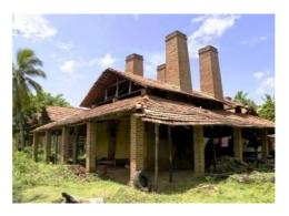
Tile factories are built up in production units. Each unit has one pug mill (to take coarse aged clay, of correct moisture content and clay blend, and to extrude finely blended, workable clay), two or more tile presses, adequate clay and tile storage, and a kiln. Some large factories will include as many as six of these units on the same site, operating for the most part independently. These units use land and labor to their utmost, and are easily managed by two site supervisors.
